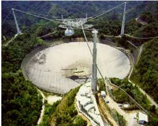
Figure 7: A spherical fixed main reflector antenna at Arecibo, Puerto Rico, USA, 305 m diameter.
