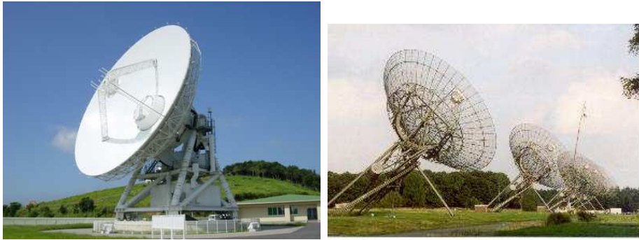
Figure 5: Alt–Azimuth mount antenna at the VERA Iriki station, Japan (Left), and Equatorial mount antennas in the WSRT, the Netherlands (Right).
