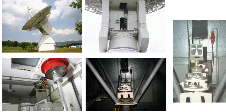
Figure 12: In 20 m geodetic VLBI antenna (Top, Left) at Wettzell, Germany, a compact receiver room is located in the back structure of the main reflector, and the Az–El cross point is covered by a cabin fixed on a rotating disk above the azimuth gear (Top, Middle). There is a firmly supported measurement bench in the cabin (Bottom, Middle). Vertical displacement of the bench is accurately monitored with respect to the invar tube which is fixed to the ground and vertically extended along the Az-axis (Bottom, Left). The target on the bench (Right) is adjusted to the right cross-point of the two axes, and is measured from geodetic markers on the ground through a hatch of the cabin (Top, Middle).
