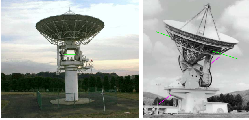
Figure 10: Alt–Azimuth mount 11 m antenna at Kashima, Japan (left), and Equatorial mount 43 m antenna at Green Bank, USA (Right). Locations of fixed and moving axes are schematically shown by straight lines.
