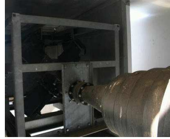
Figure 84: 2 and 8 GHz feed horn of Tsukuba 32 m antenna.
