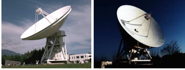
Figure 9: A flexible 45 m Millimeter-Wave Telescope at Nobeyama, Japan (left), and a “stiff” 32 m geodetic VLBI antenna at Tsukuba, Japan (Right).
